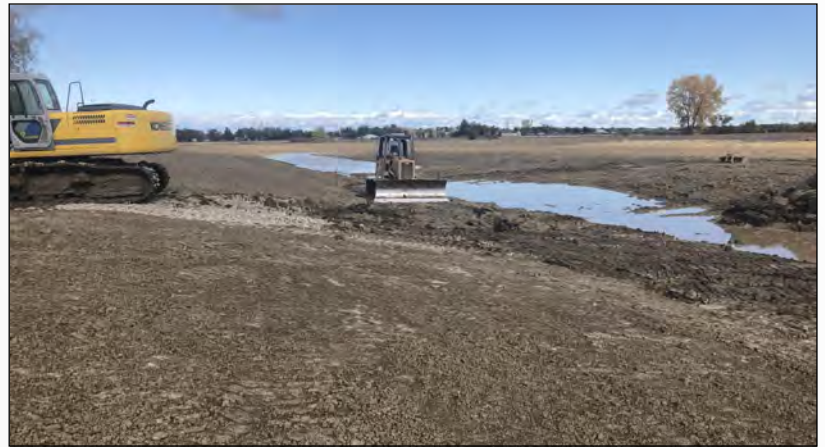
A 39 acre wetland restoration underway just south of Port Clinton.
