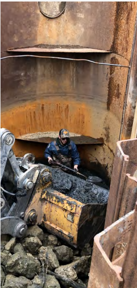
"Other duties as assigned". Wetland Tech Trevor Zook cleaning sediment from the MS 8b pump intake pipe.
